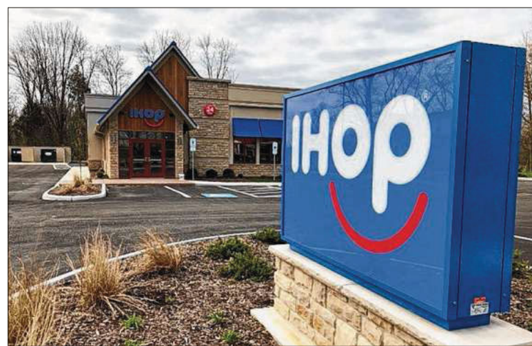
The IHOP restaurant at 3324 Benchwood Road near the Miller Lane/York Commons development in Vandalia is all revved up and ready to go, but it still has not opened. MARK FISHER/STAFF
