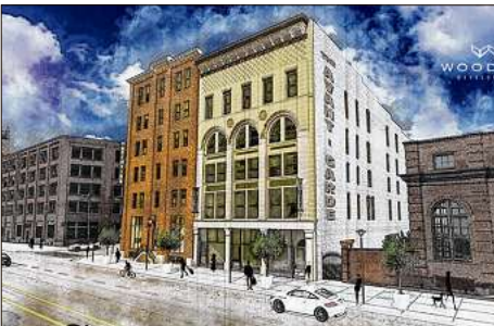
The old Lotz paper building at 607 E. Third St., renamed the Avant-Garde, is the home of Tangram Flex. CONTRIBUTED
